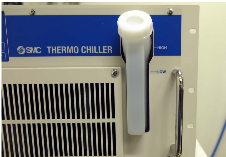
Figure 34. Coolant filling and coolant level locations for the SMC chillers
