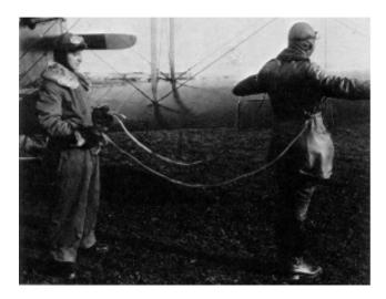
Figure 3.13 A bombardier and pilot demonstrate the signaling reins used to communicate turn commands during a bomb run.<sup>110</sup>
